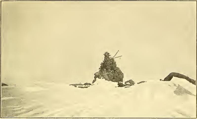
BEACON BUILT ON BELL ISLAND.
