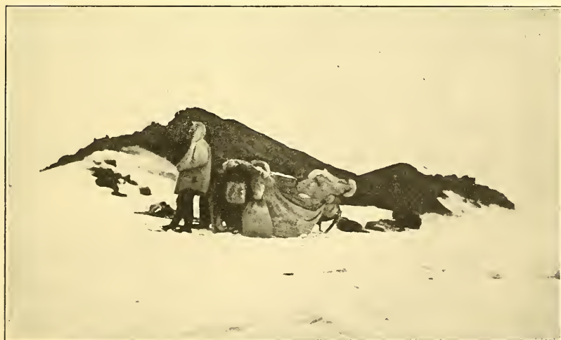
ONE METHOD OF FORMATION OF UNDERGROUND ICE. A dagger of ice is stabbed into bank and broken off, leaving ice covered by a heap of dirt.
